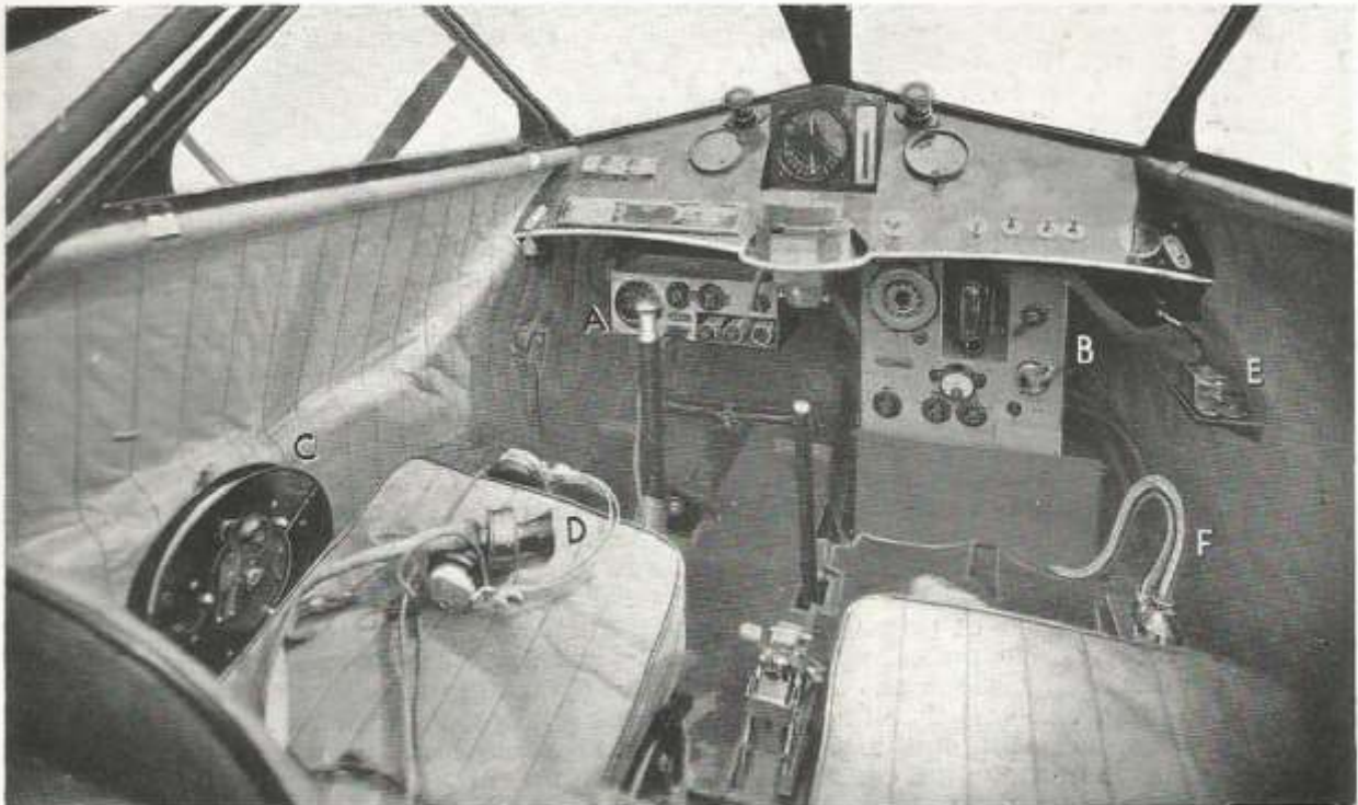
MARCONI TYPE AD 49/50 MEDIUM WAVE AIRCRAFT TRANSMITTING AND RECEIVING EQUIPMENT INSTALLED IN A MONOSPAR TYPE ST4
