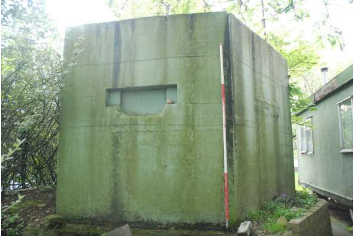
Illus 112 Pillbox Structure 41 north-facing elevation with blocked embrasure
