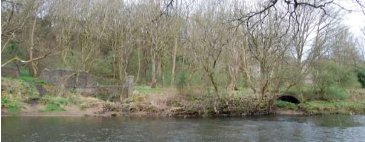
Illus 100 Culvert S10 (right) and S33 (left) with S34 between from north bank of river Don; facing SW
