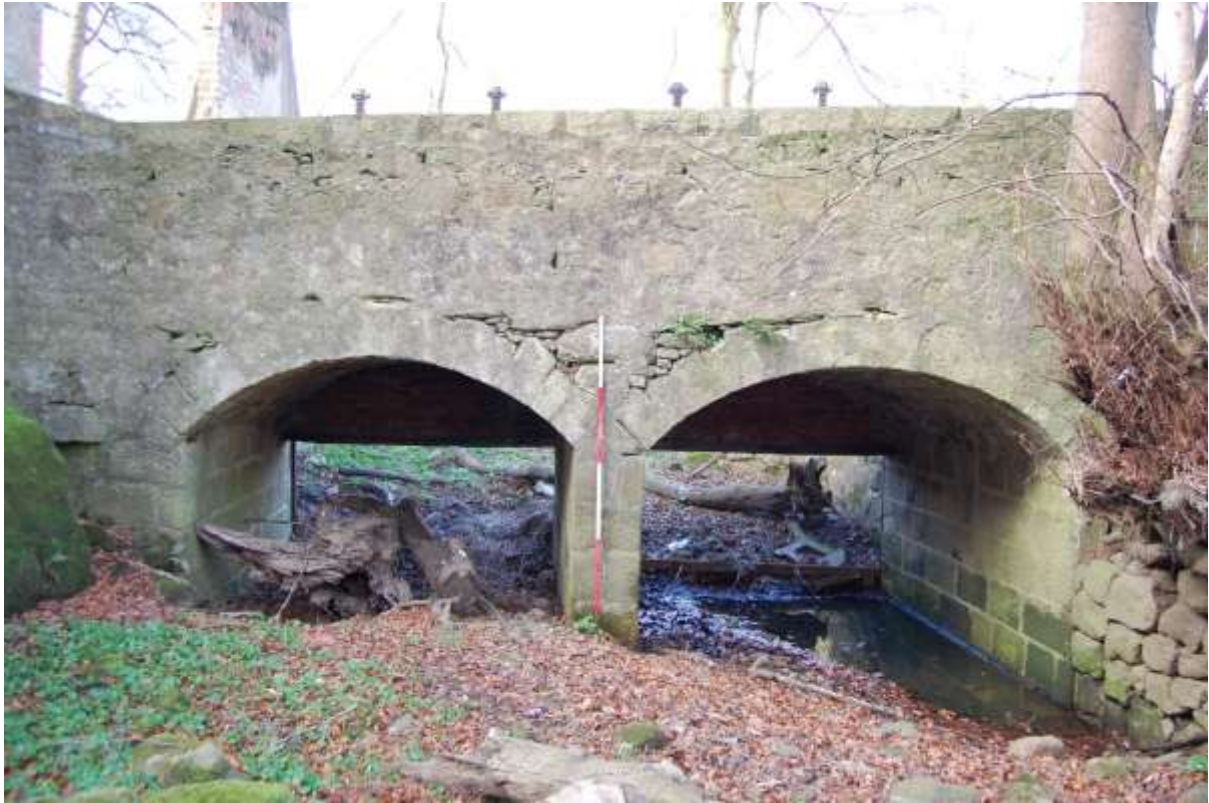
Illus 56 Bridge S15 over Lade S6; facing SW
