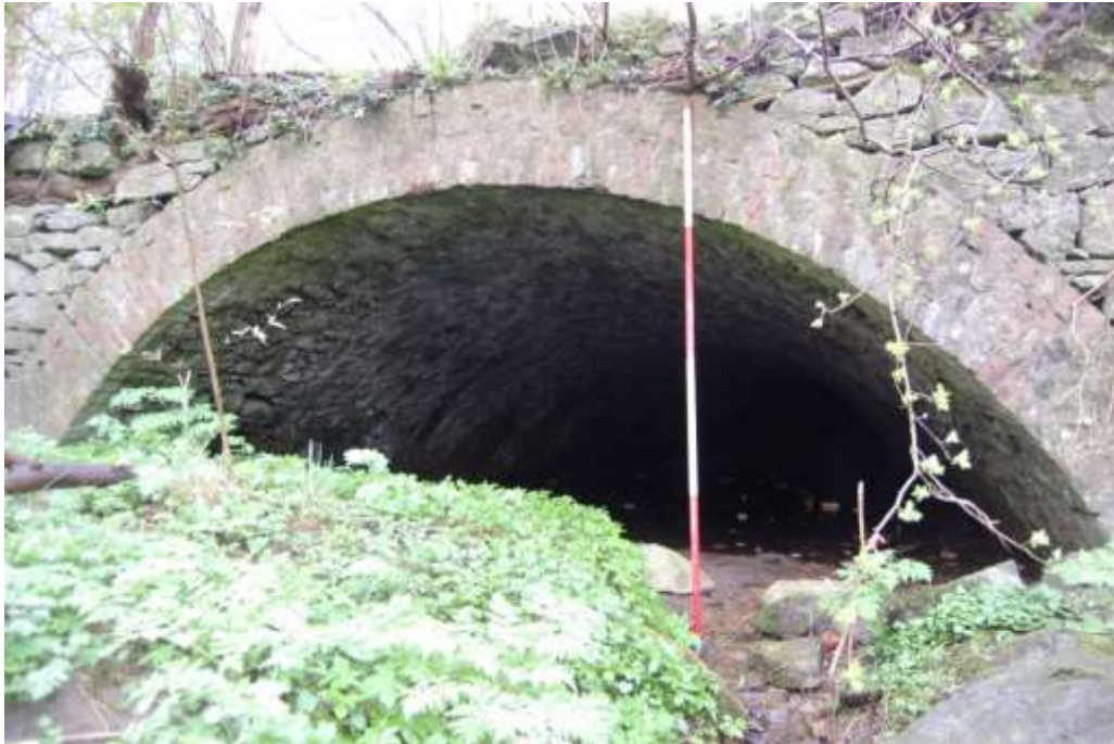
Illus 43 Culvert S10 at outflow into river Don; facing SW
