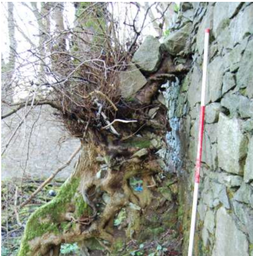
Illus 49 Buttress on the interior of the south wall of enclosure S11 showing damage from trees
