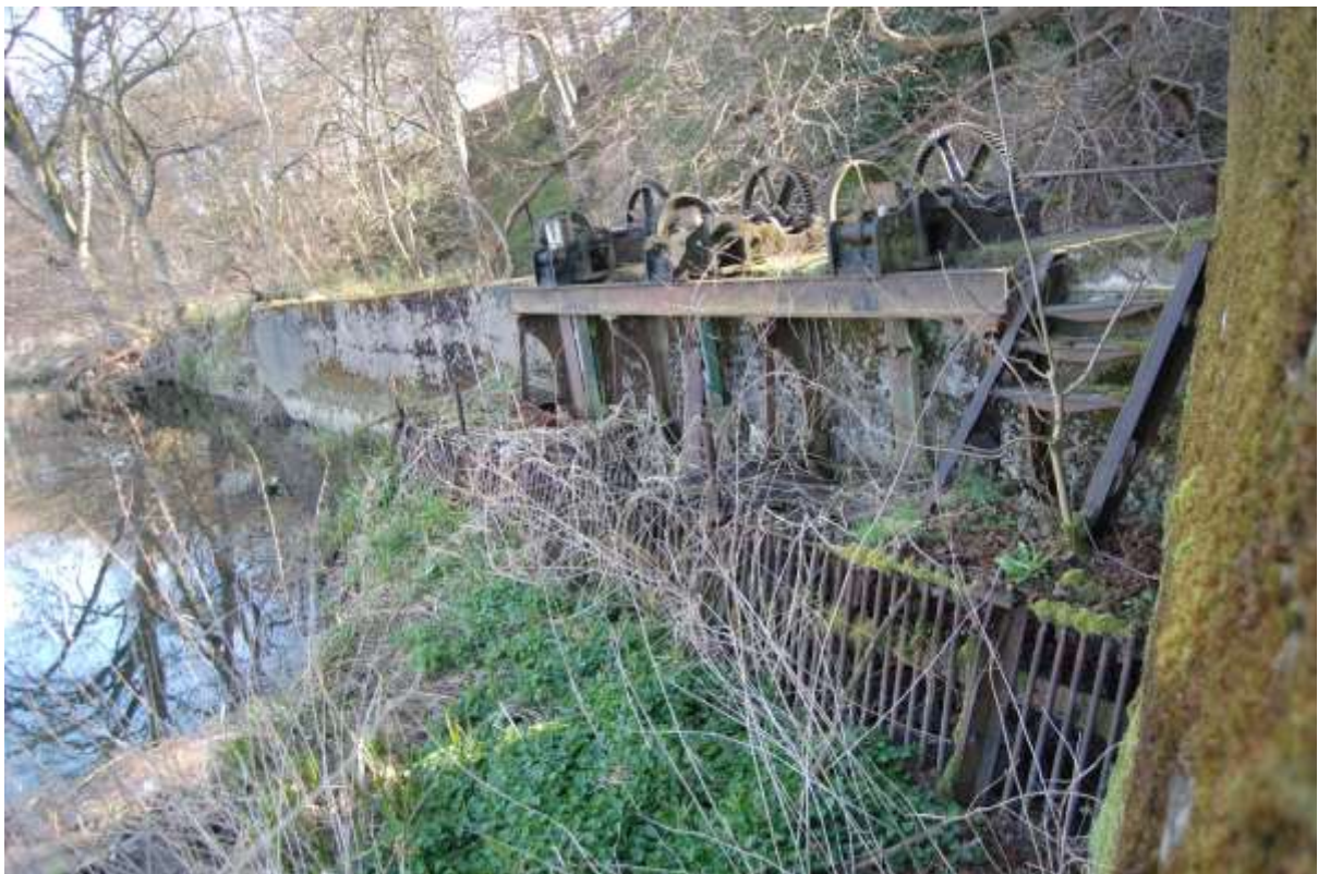
Illus 89 S27 sluice mechanism; facing E
