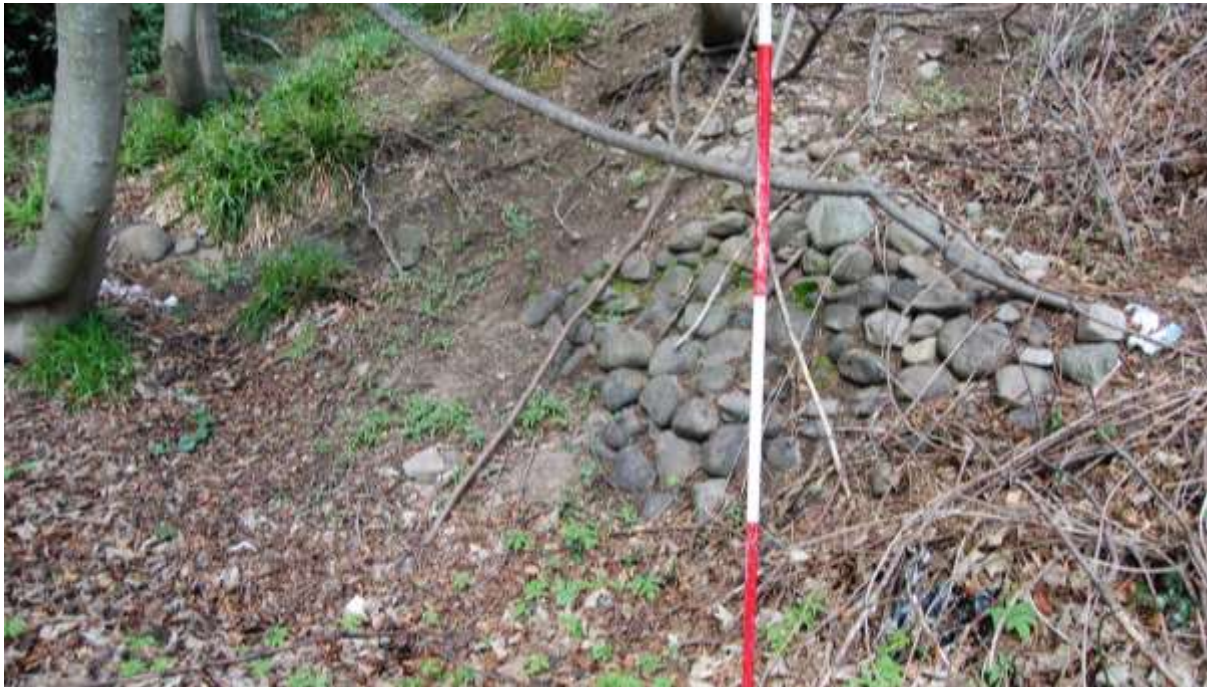
Illus 110 Stone revetment S39 on south side of mound S40; facing NE
