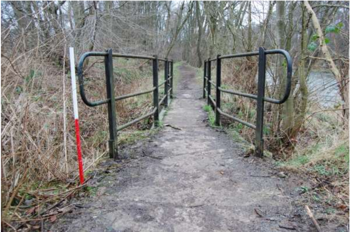
Illus 91 The bridge S28 facing west
