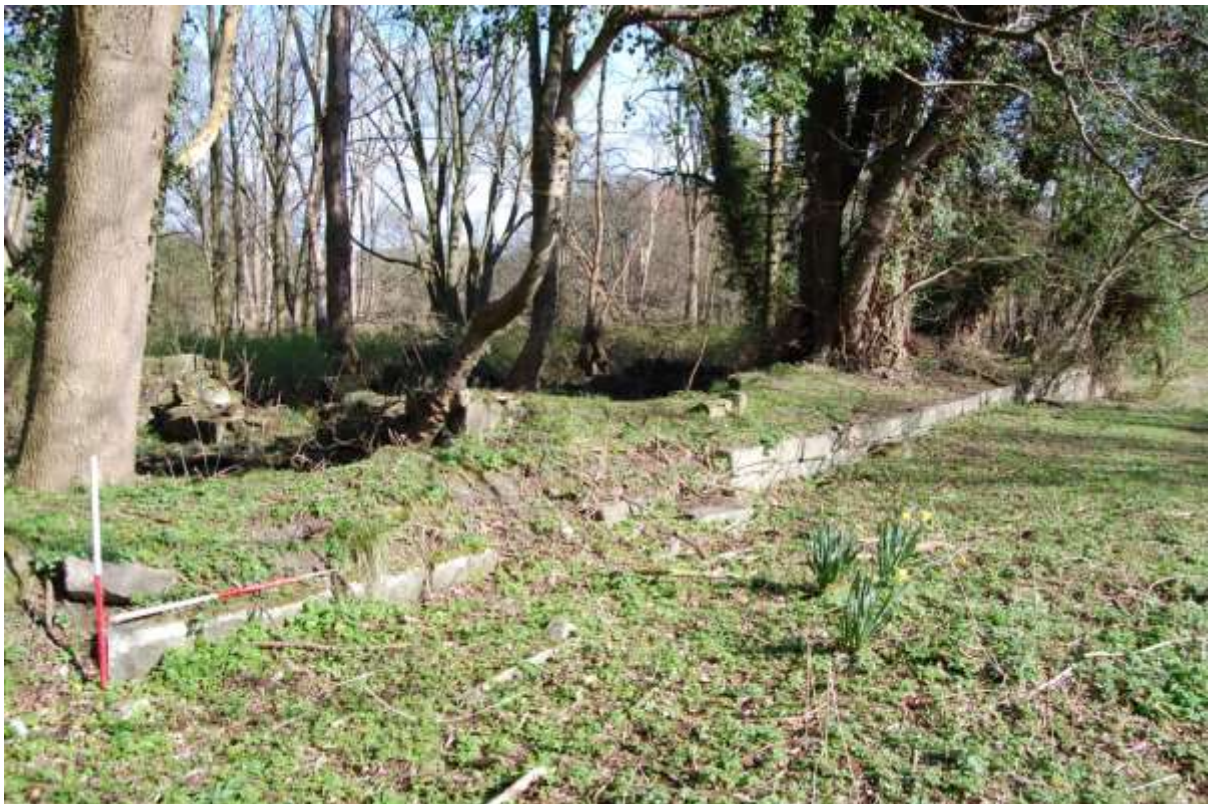
Illus 21 North wall of lade S6; the lade has been infilled (foreground)
