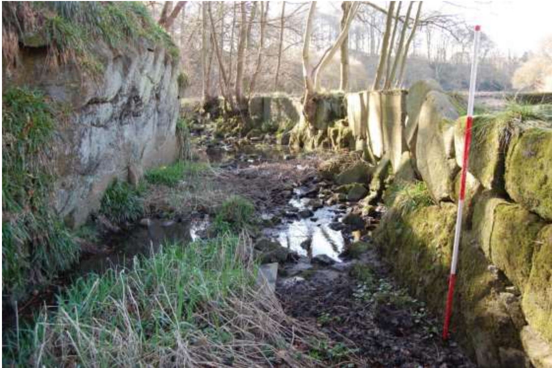
Illus 33 S6 SW of bridge and sluice S14; facing SW
