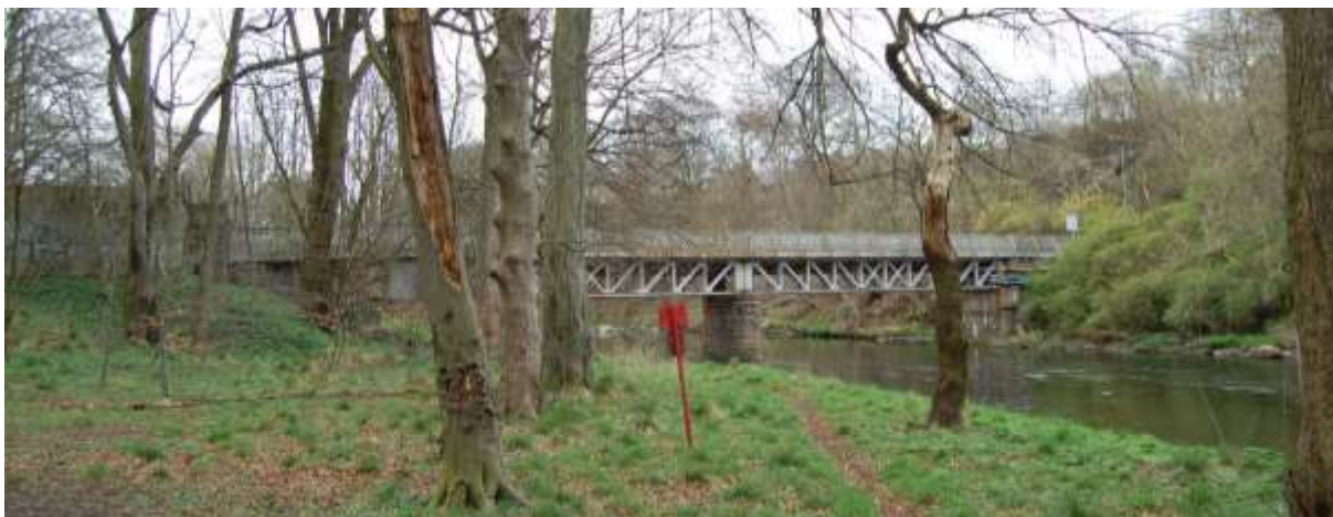
Illus 118 Grandholm foot bridge; facing E
