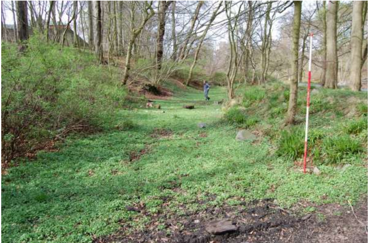
Illus 29 Lade S6 adjacent to Woodside House (left) partly infilled; facing W
