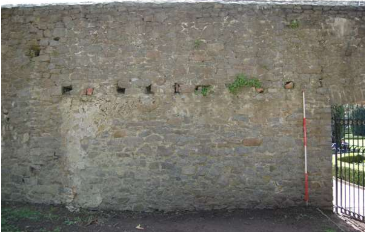
Illus 72 Joist holes from demolished building on exterior of north wall of walled garden S19; facing S
