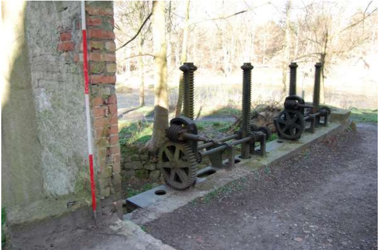
Illus 54 Sluice gate mechanisms on the west side of the bridge
