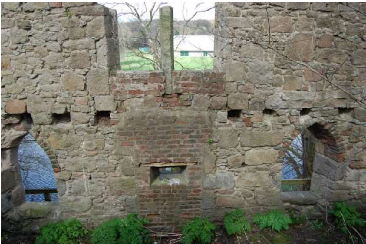
Illus 65 Structure 16 interior of north wall showing blocked window (above) and door (below) with loophole; facing N
