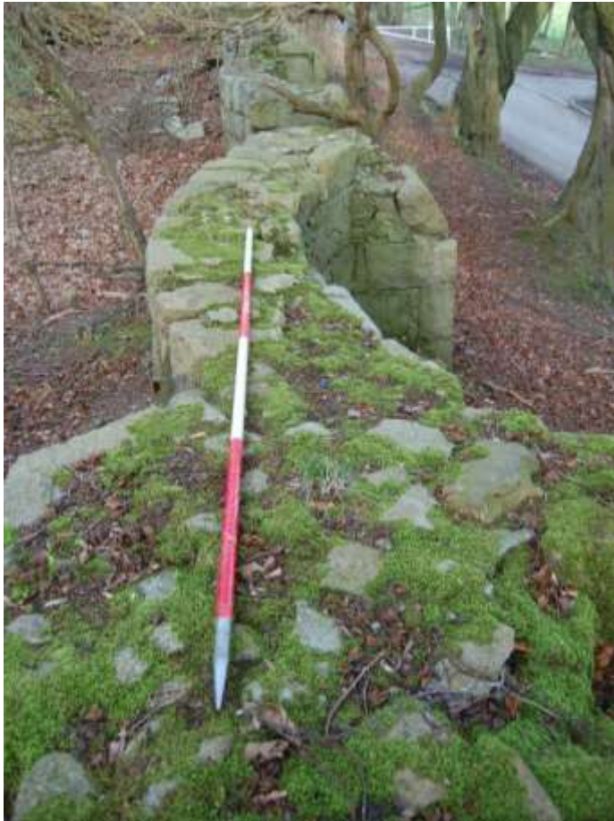
Illus 5 Structure 1 showing sections of convex curving wall between buttresses; facing ENE
