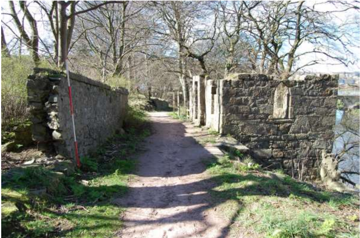
Illus 63 Building S16 (right), track and remains of boundary wall S20 (right); facing W
