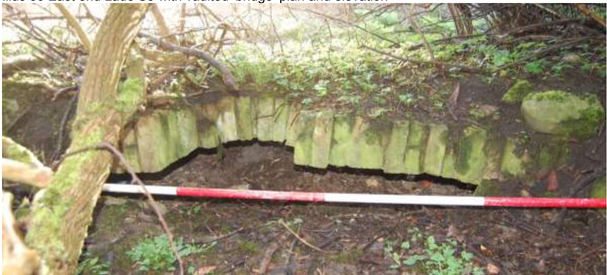
Illus 37 West side of brick vaulted 'bridge'; for location see Illus 36
