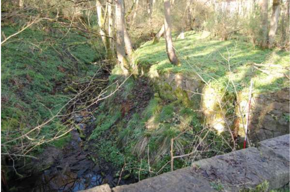
Illus 51 Lade S13 from bridge S33; facing WSW
