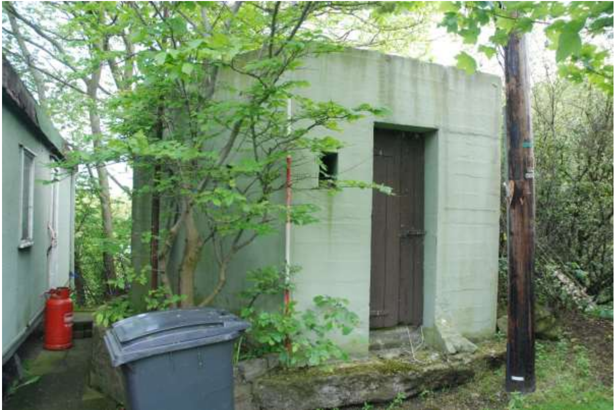
Illus 113 Pillbox Structure 41 south facing external wall showing central door, small aperture and 30cm thick concrete foundation
