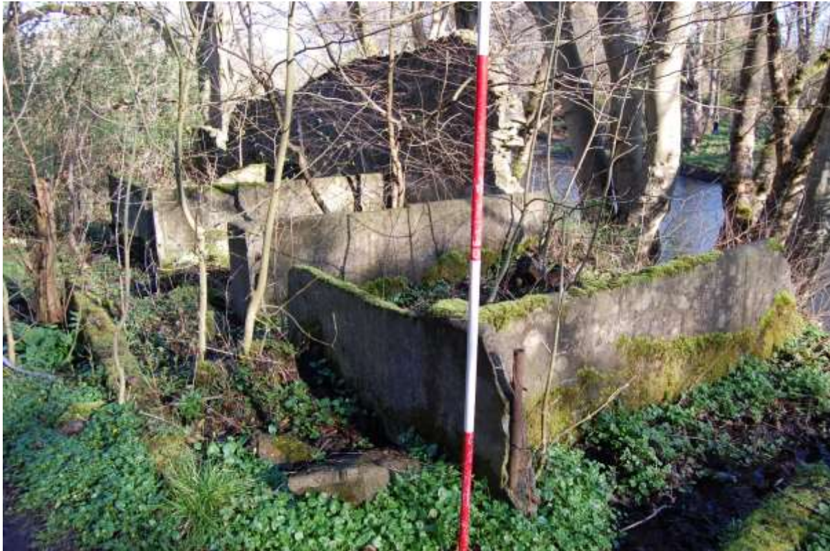
Illus 50 Structure 12 showing concrete partitions in older granite building
