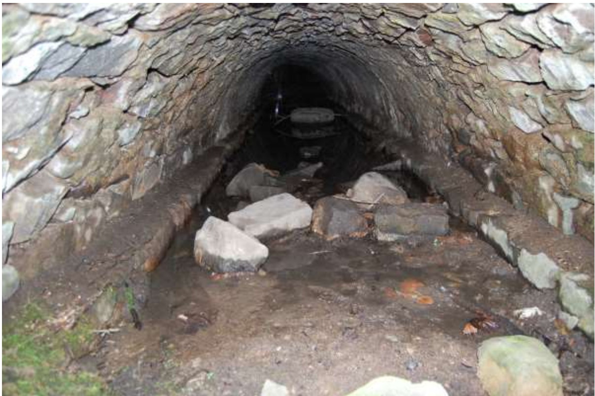
Illus 105 Culvert S36 showing stone vaulting on stone foundation; facing NW
