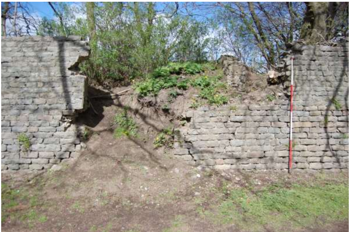
Illus 71 Wall S21 with wall of S17 (left of ranging rod) showing poor condition of walls and overgrown and infilled structure with remains of entrance (left of centre)
