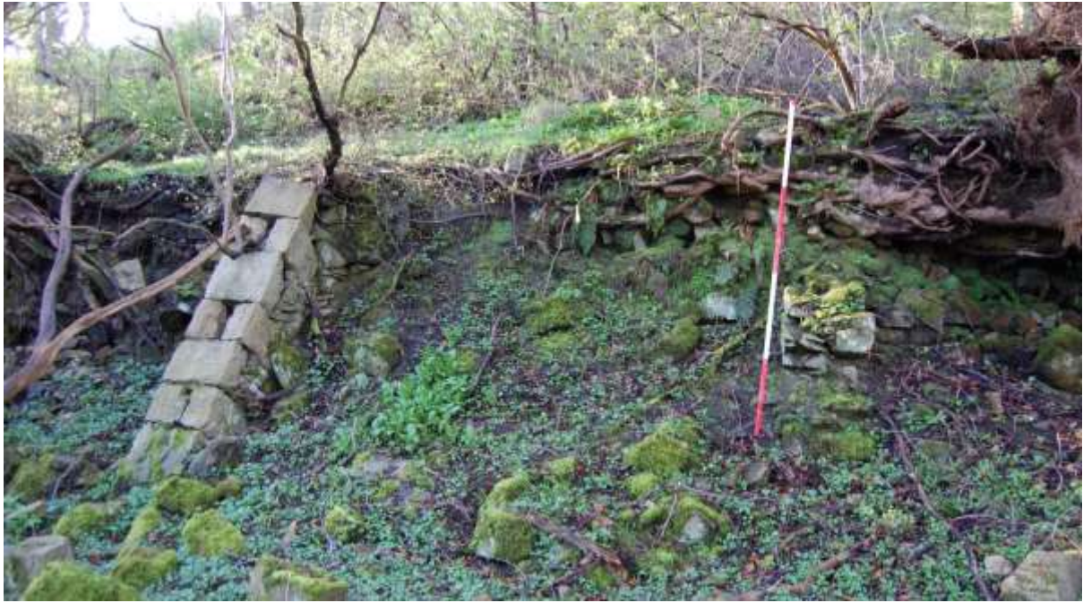
Illus 48 Buttresses on the interior of the south wall of enclosure S11
