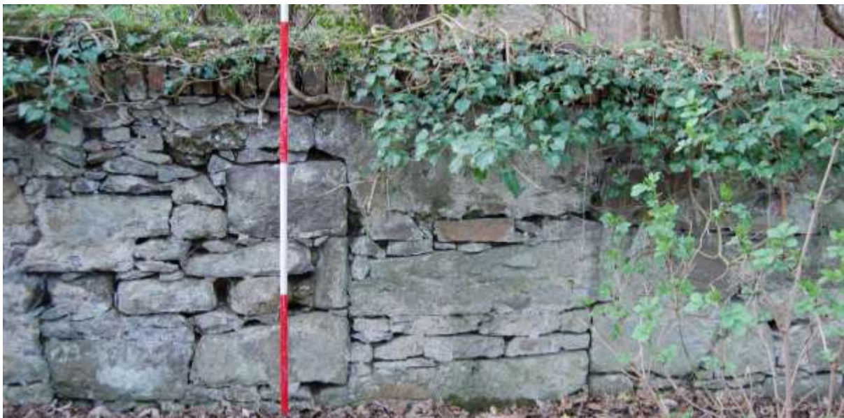
Illus 26 North façade of north wall of lade S6 showing one of the inserts of masonry
