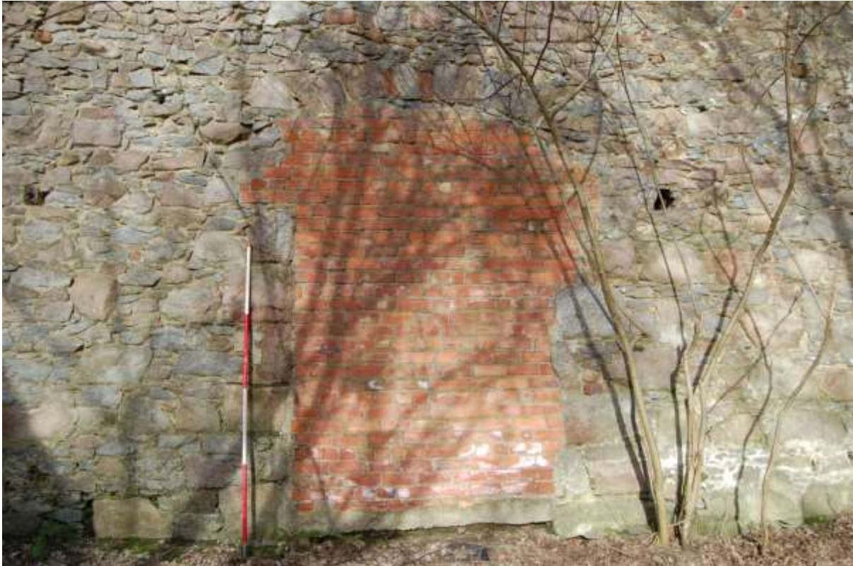
Illus 13 Structure 3 west gable interior face showing blocked door; facing W
