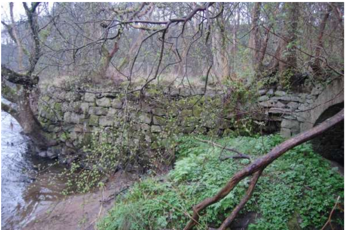
Illus 101 Stone embankment S34 (centre) with culvert S10 (right)
