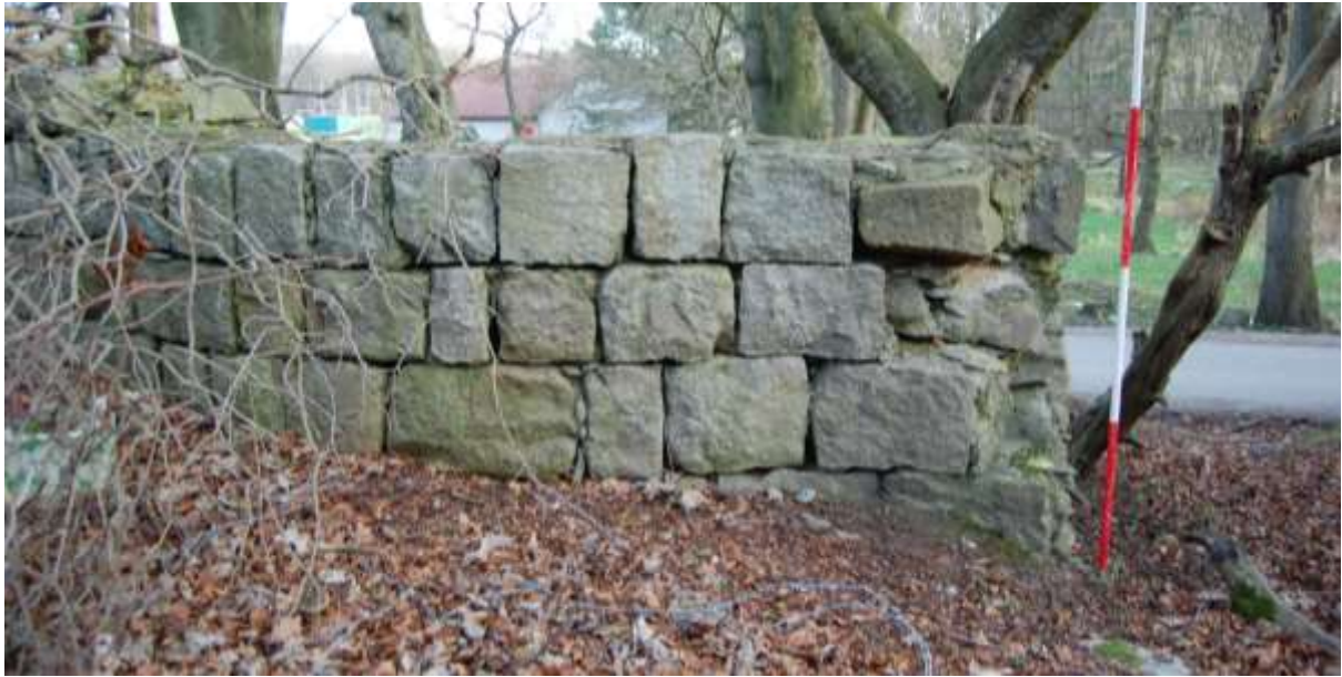
Illus 7 Structure 1 south (inner) face of wall; facing N
