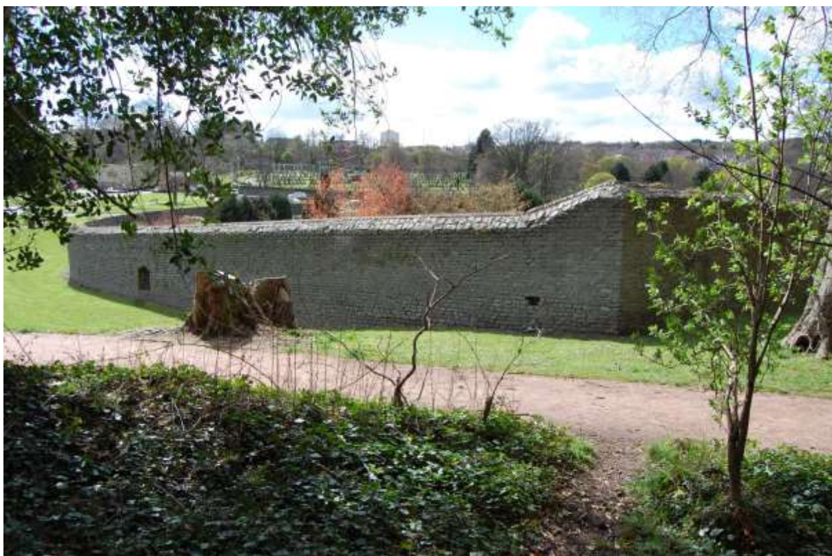
Illus 74 Walled garden S19 showing thicker wall on north half of garden formed using brick on the interior; facing SW
