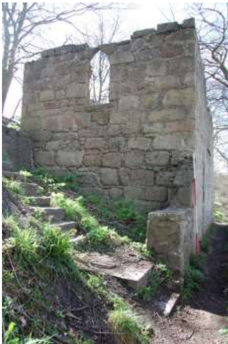
Illus 67 Structure 16 east wall showing structure built into the slope and the narrow path adjacent to the slope down to the river (right); facing WSW
