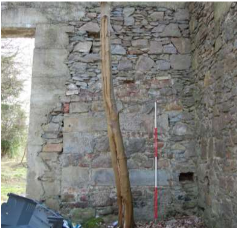
Illus 14 Structure 3 east gable interior face showing blocked doorway on south side of the newer larger central door; facing E
