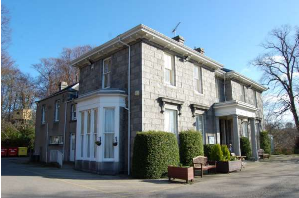
Illus 84 South façade (right) of Woodside House; facing NE
