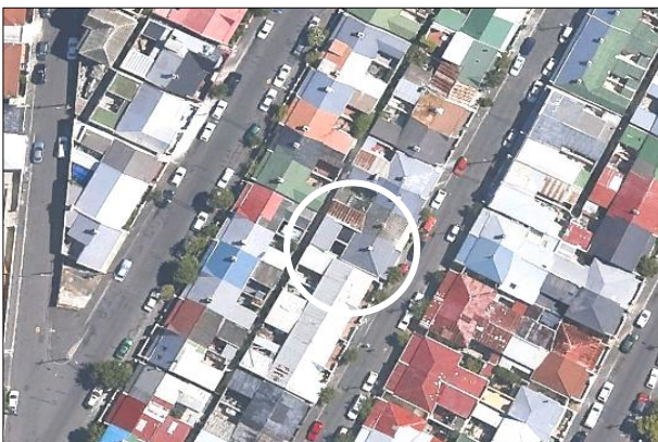
Figure 11. Aerial view showing urban context of row housing, with building circled.
