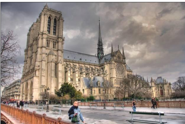
Figure 3. The Gothic Cathedral of Notre Dame in Paris was as a sign of wealth and pride in twelfth century Europe, and achieved greater heights by means of pointed arches and flying buttresses. ( http://opentravel.com/notre-dame-cathedral-cathedrale-de-notre-dame-de-paris-paris-france ).
