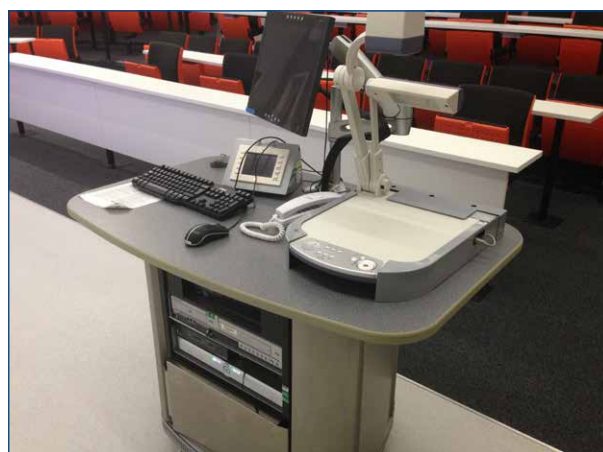
Photo 11: AV pods in the interactive lecture theatres at City University are equipped with a range of learning technologies including: visualiser, interactive pen and digital flipchart.
