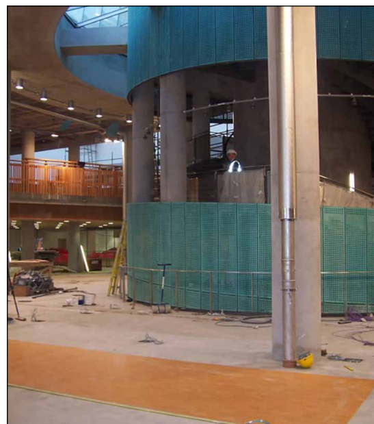
Photo 4: Construction work at the Saltire Centre, Glasgow Caledonian University.
