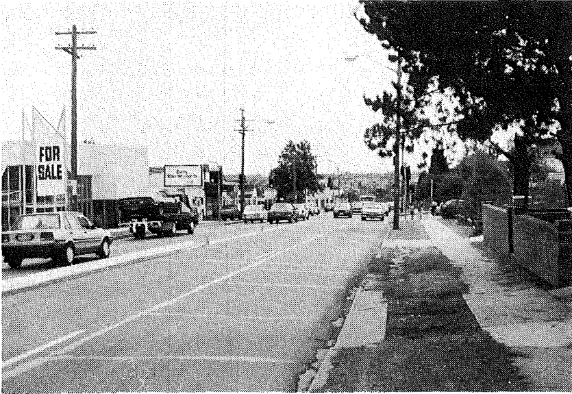
Figure 1: Lack of sheltered right turn bays reduce available through lanes on Canterbury Road, Punchbowl.
