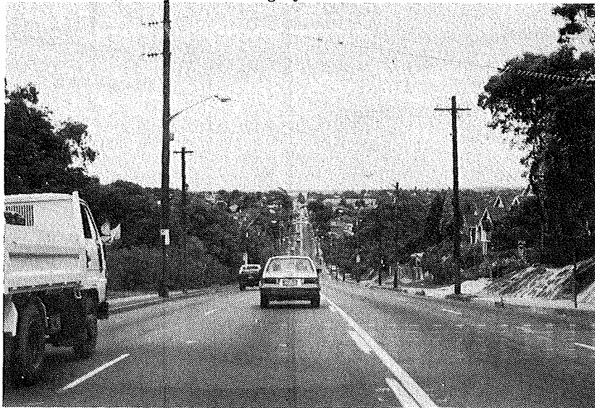
Figure 9: King Georges Road is constructed over a series of short, steep sections thereby reducing visibility.
