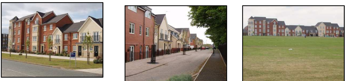
Figure 5.12 a&b: Images of Westoe Crown Village development
