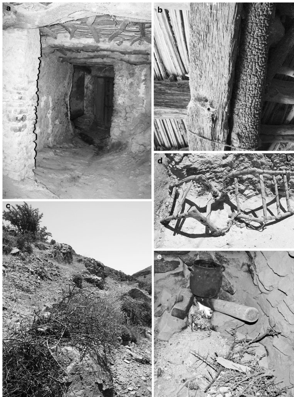
Fig. 10 Uses of Argan tree at Tifigit; a joist of roof; b date palm ( left ) and argan tree ( right ) timber as beams; c spiny branches for fencing; d packsaddle frame of argan wood (mule); e argan twigs as domestic fuel (Tifigit, photographs Ruas/Tengberg, April–May 2009)
