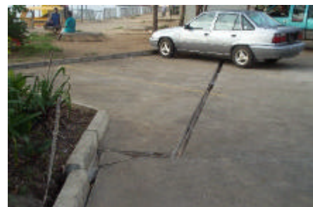
Figure 9: Car park slabs opened south of Market
