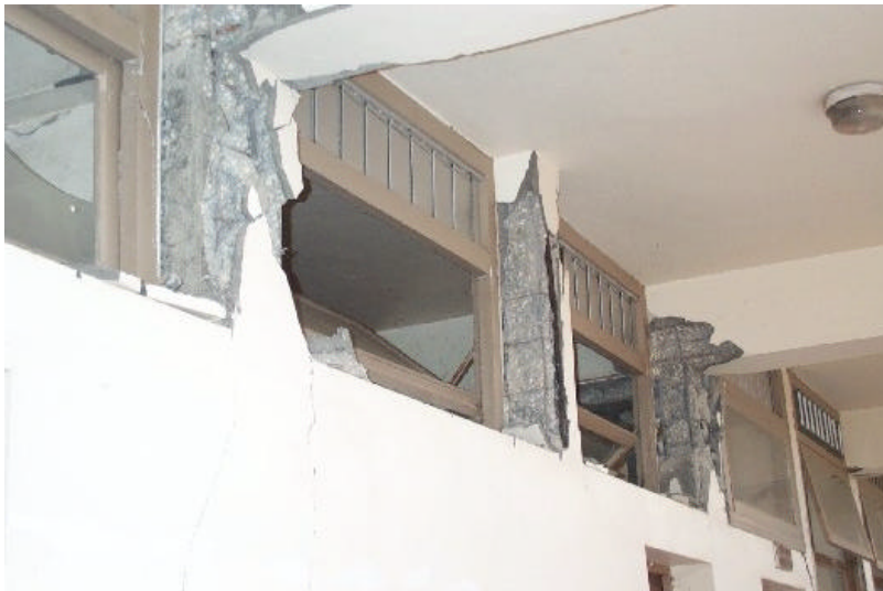
Figure 4: Short columns spalled and failed, ground floor, Lycee Bouganville
