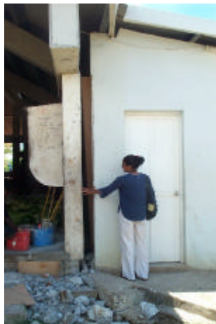
Figure 8: Detached Market toilet block
