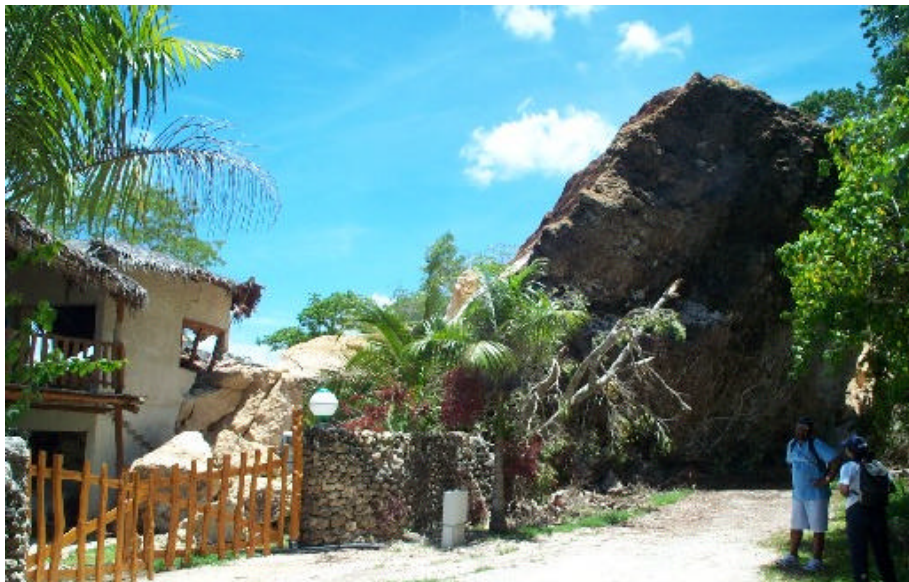
Figure 19: Toppling failure from the cliff face behind Pango Resort
