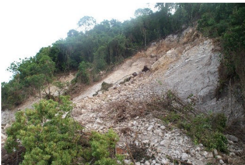
Figure 16: Massive slope failure in tuff above Wharf access road
