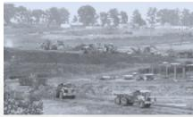
Designed to span I-285, the runway project required moving more than 18 million cubic yards of earth fill from offsite borrow pits by means of a 5.5-mile long conveyor belt and discharge bin system, and the construction of a full-length parallel taxiway and dual north/south taxiways.
